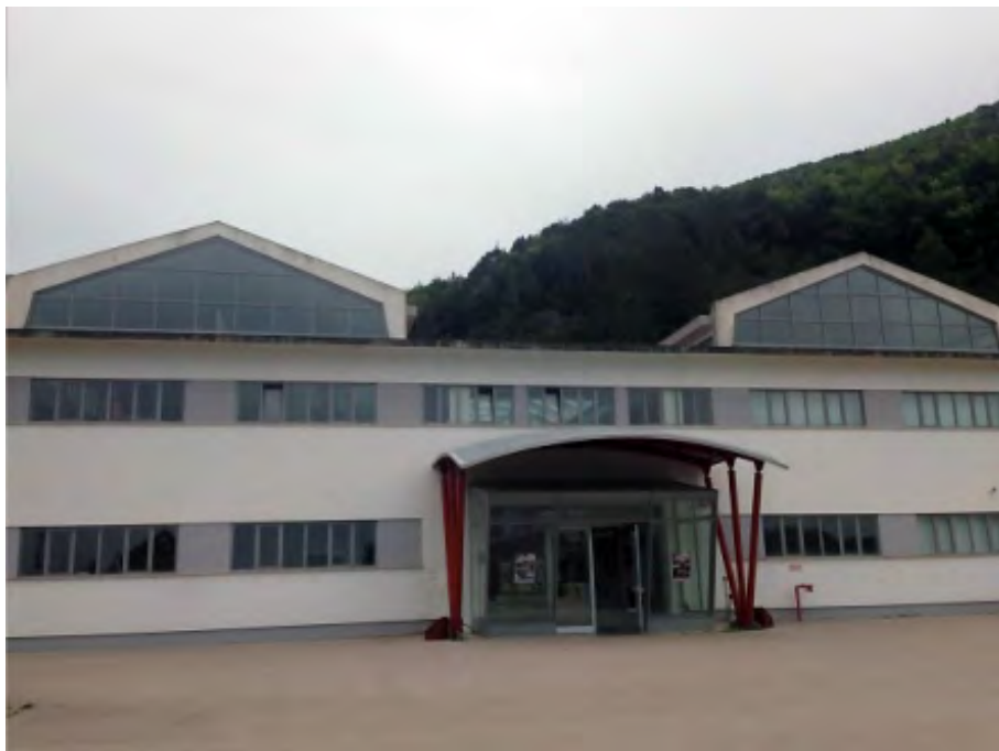
Figure 14. Roofed gallery and new entrance after the restoration.
