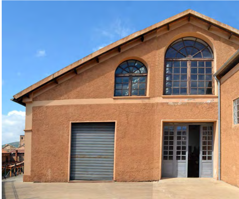
Figure 28. The east facing today: the arched window on the right was removed from the volume set against the engine room. Photo by the author.
