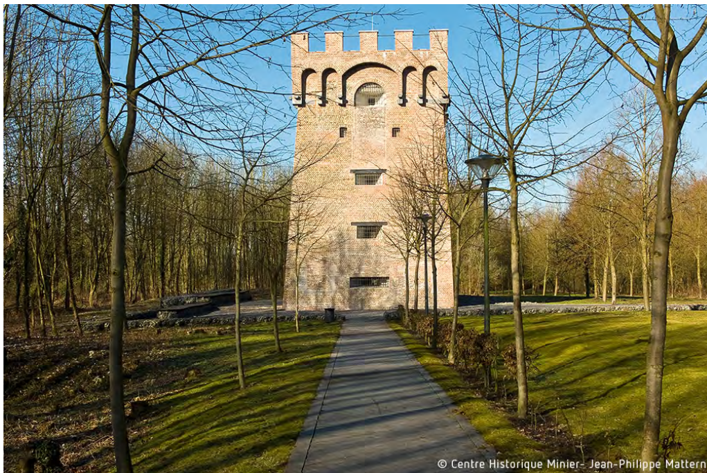
Figure 20. The Sarteau fire station. Source: www.bassinminier-patrimoine mondial.org
