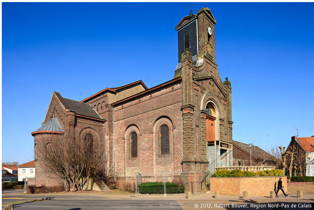
Figure 29. Church of Saint Barbara, former the Shaft of la Sentinelle. Source: www.bassinminier-patrimoine mondial.org
