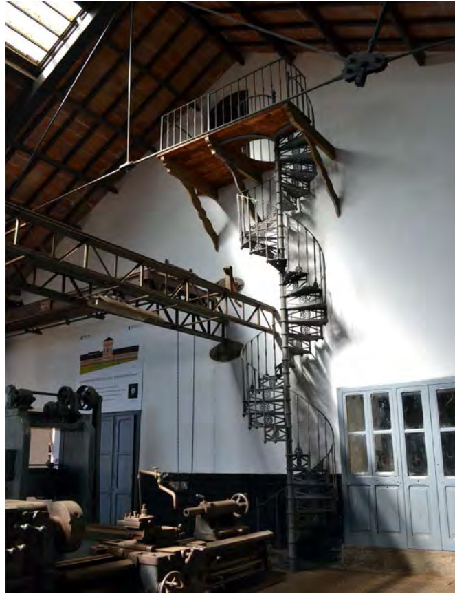
Figure 14. The cast iron staircase connecting the engine room to carpentry. Photo by the author.
