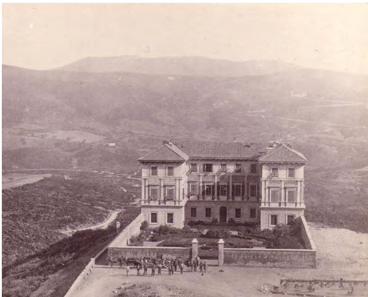
Figure 5 Directorate and Manager's house "Bellavista" in 1866 5 . Source: Archive IGEA Spa.
