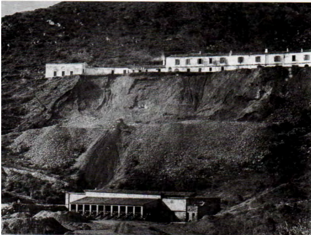
Figure 2. The Saint Real washery and up the St. Vittorio yard. Source: Ottelli, L. (2010).
