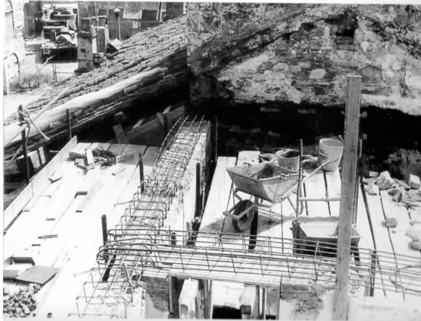
Figure 5. Reinforcement and restoring interventions of the oofs. Source: Franchina, L., 1998.
