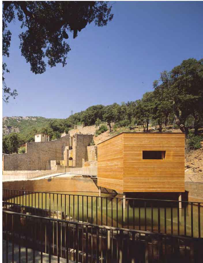
Figure 10. A view of the Dorr. Source: Pieri, E. Costruire in Laterizio 99, 2004.
