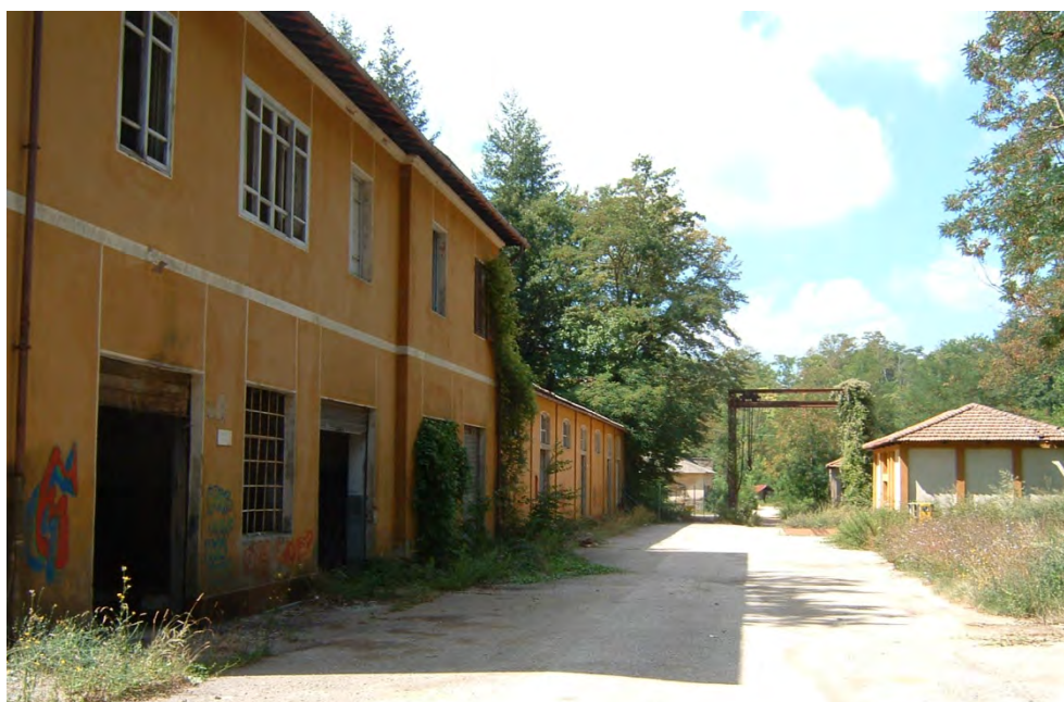
Figure 17. The archives before the restoration. Source: www.massacomune.it e www.ilgiunco.net
