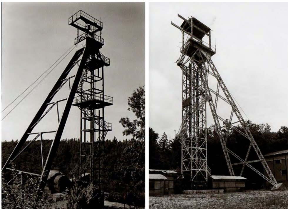
Figure 8. On the left Tosi shaft, on the right Rostan shaft. Source: Preite, Paesaggi industriali del Novecento , 2006.
