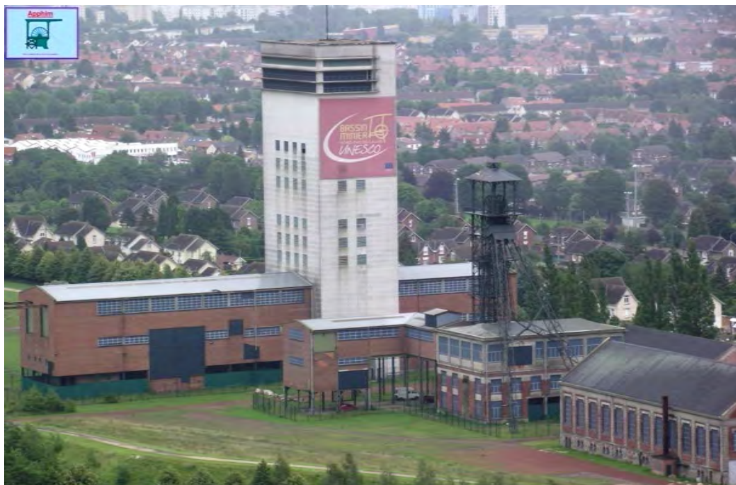
Figure 34. The complex of 11/19 Shaft today. Source: www.bassinminier-patrimoine mondial.org
