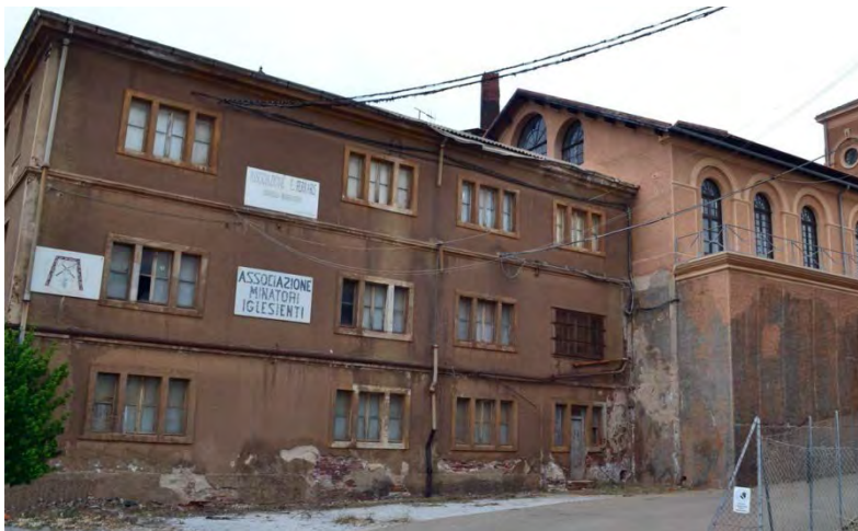
Figure 25. The Association's Building E. Ferraris today. Photo by the author.
