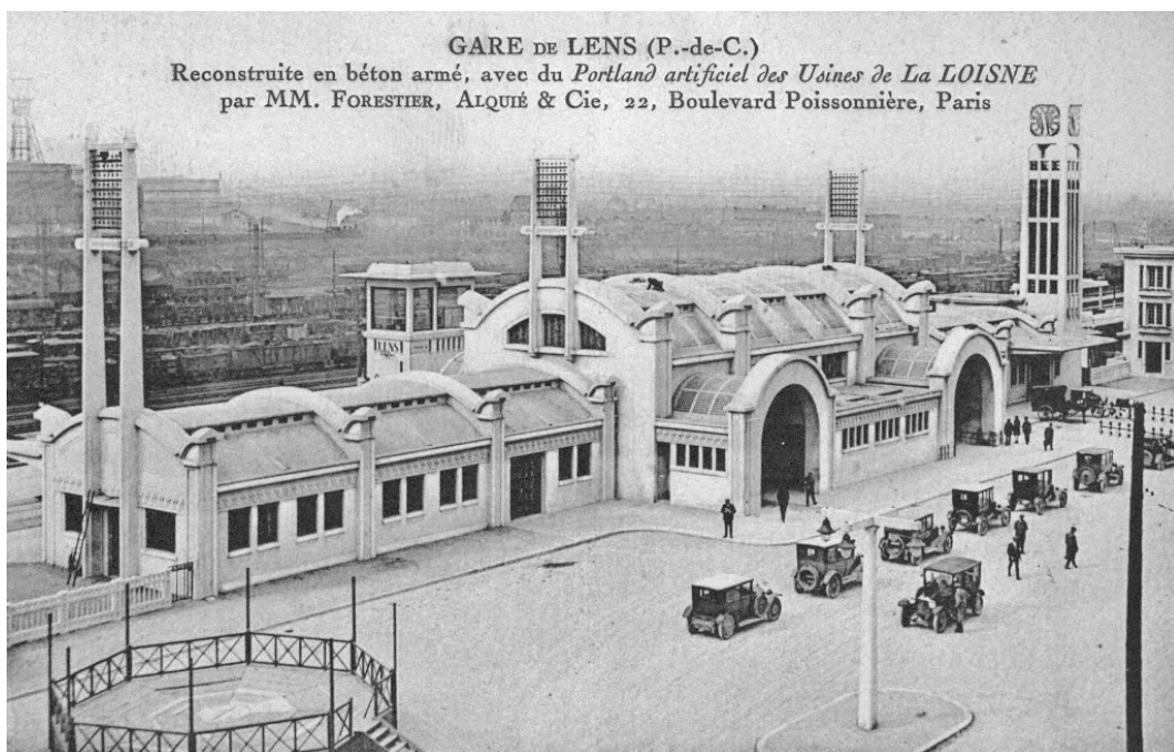
Figure 23. Lens Station after the reconstruction. Source: www.cdclens.fr/cp-gare-depot.html
