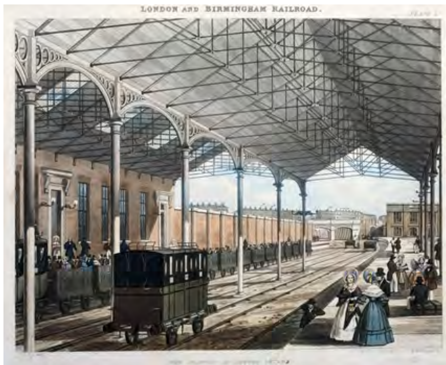
Figure 20 Euston Station in London. Source: http://lowres-picturecabinet.com .
