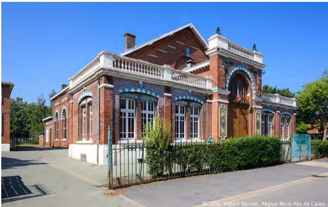
Figure 12. Hall of Parties of the Cité d'Arenberg. Source: www.bassinminier-patrimoine mondial.org
