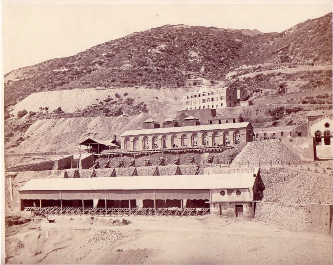
Figure 11. The Vittorio Emanuele manual Washery around 1875. Source: Archive IGEA Spa.
