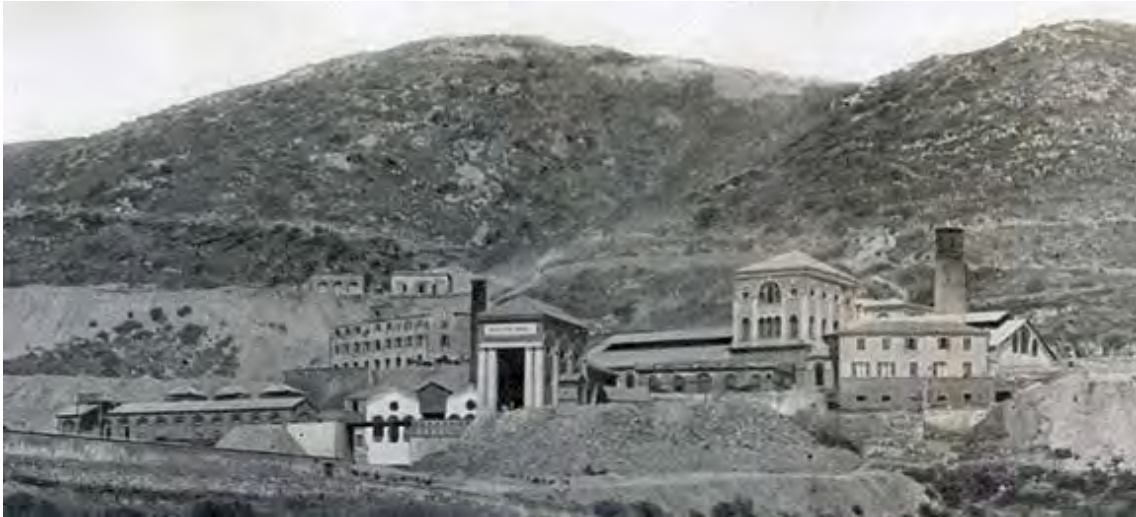
Figure 1. 1875: the skylights are present in both of the side halls. Source: Monteponi Company 1850 -1950.
