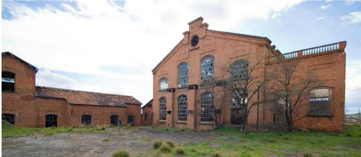
Figure 13. The Thermoelectric power station before the restoration. Source: Javier Callejas on Google Earth.
