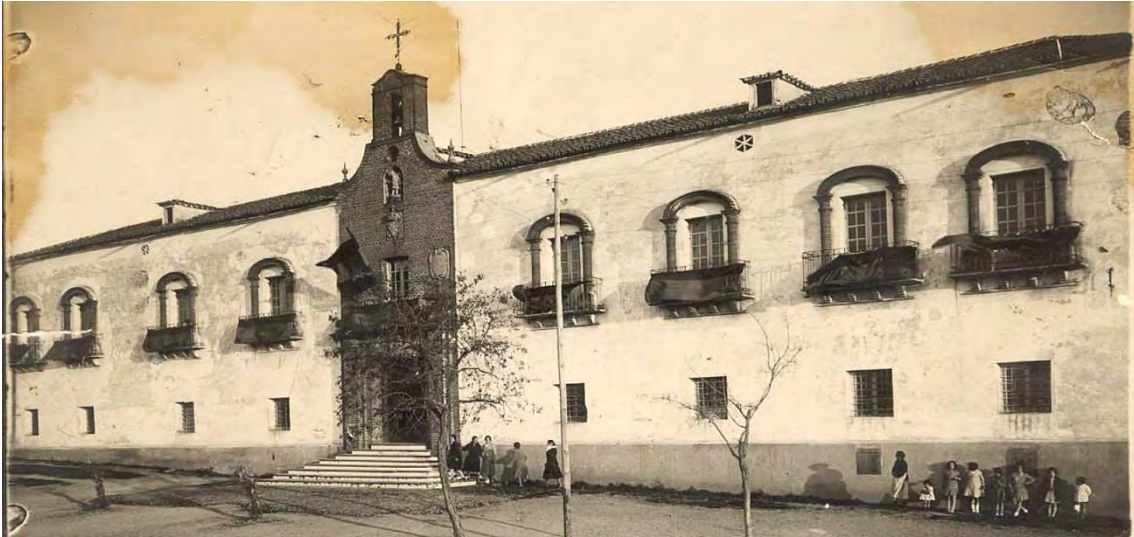
Figure 21. The Real Hospital de Mineros de San Rafael in an historical photo.
