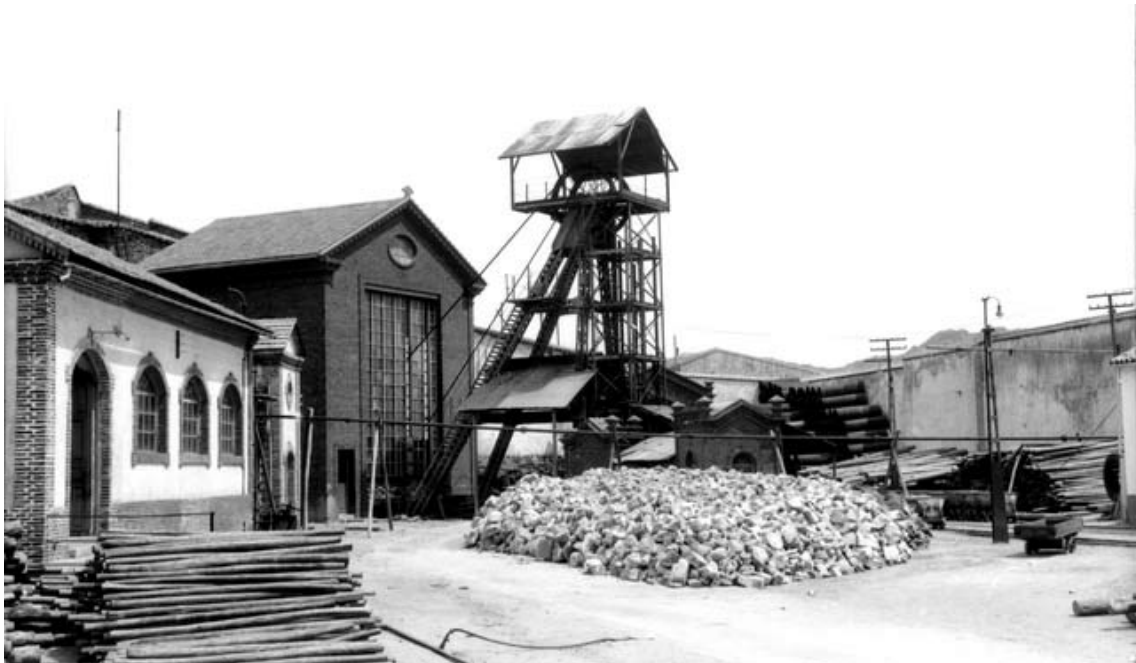
Figure 4. San Teodoro pit before the modification in 1962. Source: mti-minas-castillalamancha.blogspot.it
