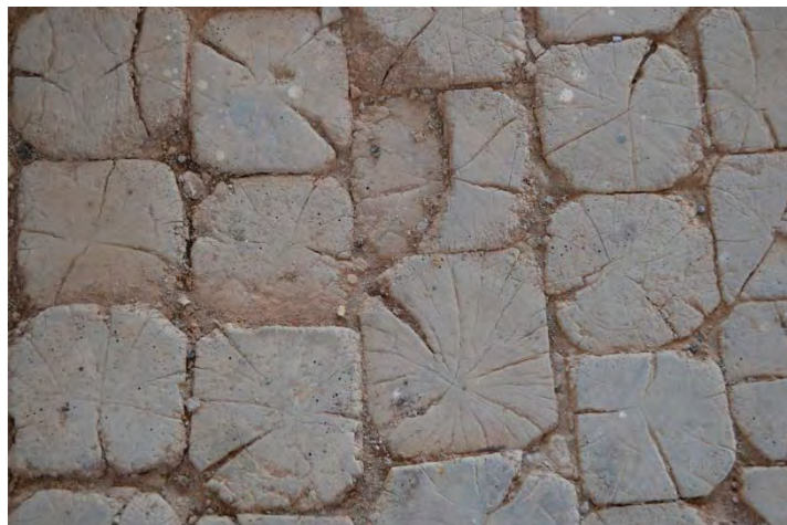
Figure 20. The floor in the wooden dowels in the added volume of the carpentry. Photo by the author.
