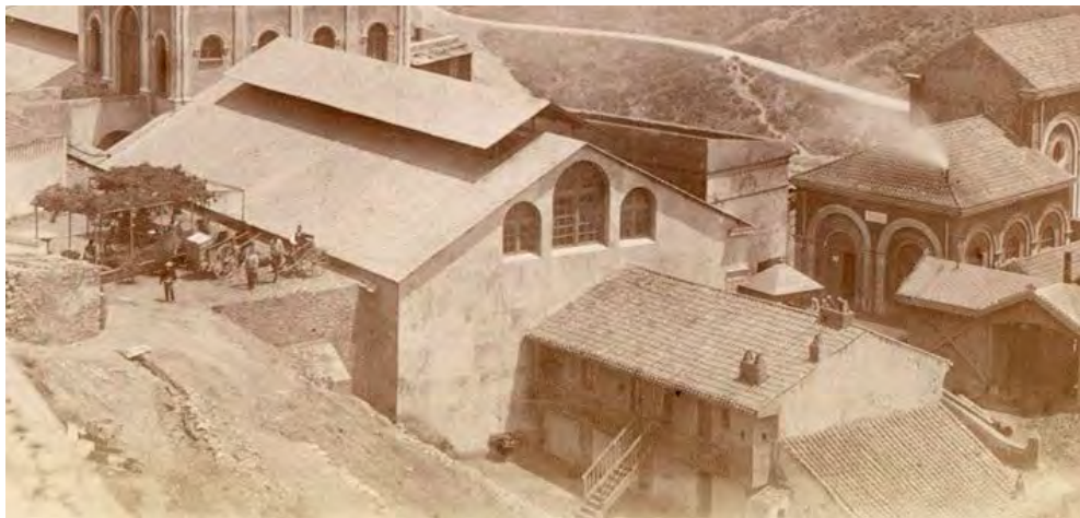
Figure 22. The building with the stairs of the embankment and the balcony; bottom right the single pitch coverage orthogonal to the building. Source:
