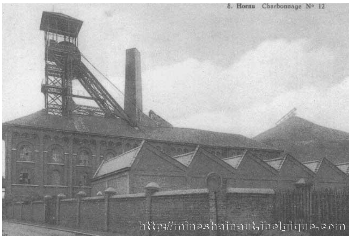
Figure 6 Lateral view of the pit. Source: http://les-charbonnages-borains.skynetblogs.be/hornu/
