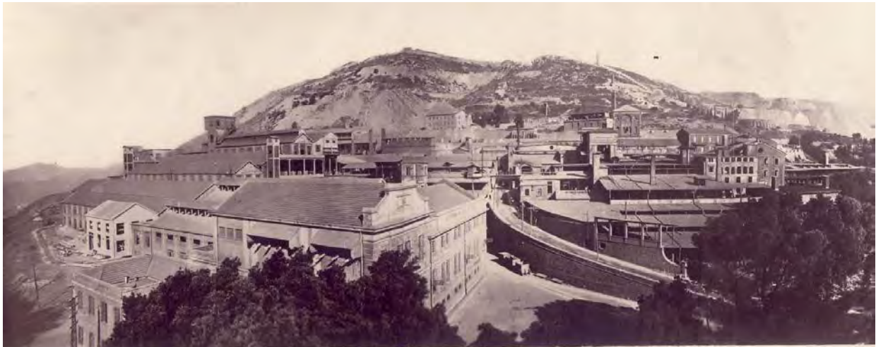
Figure 14 The electrolysis building in the foreground just realized in 1926. Source: ASCI.
