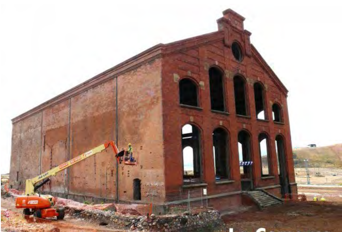
Figure 16. The external during the works of the company Sacyr. Source: https://minasdepueblonuevodelterrible.jimdo.com
