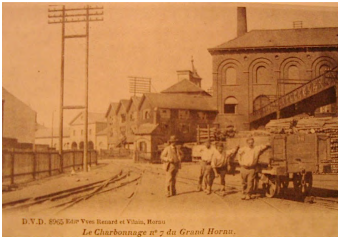
Figure 30 External view of Shaft n. 7 in Grand – Hornu. Source: http://les-charbonnages-borains.skynetblogs.be/hornu/
