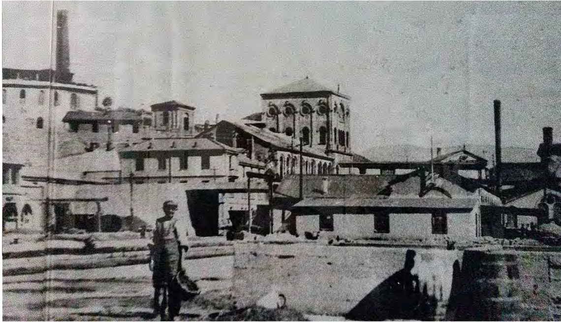
Figure 3. 1917 (?): The skylight is absent also in the left room. Photo by the author of a photo in the seat of the Sardinian Mining Association in Iglesias.
