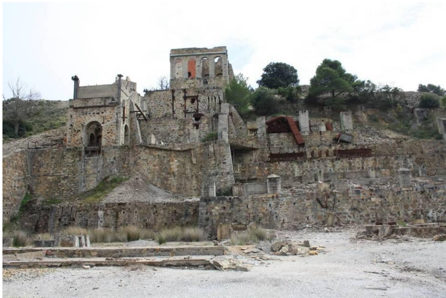
Figure 9. Ruins of the Pireddu treatment plant at Ingurtosu established in the 1920s.
