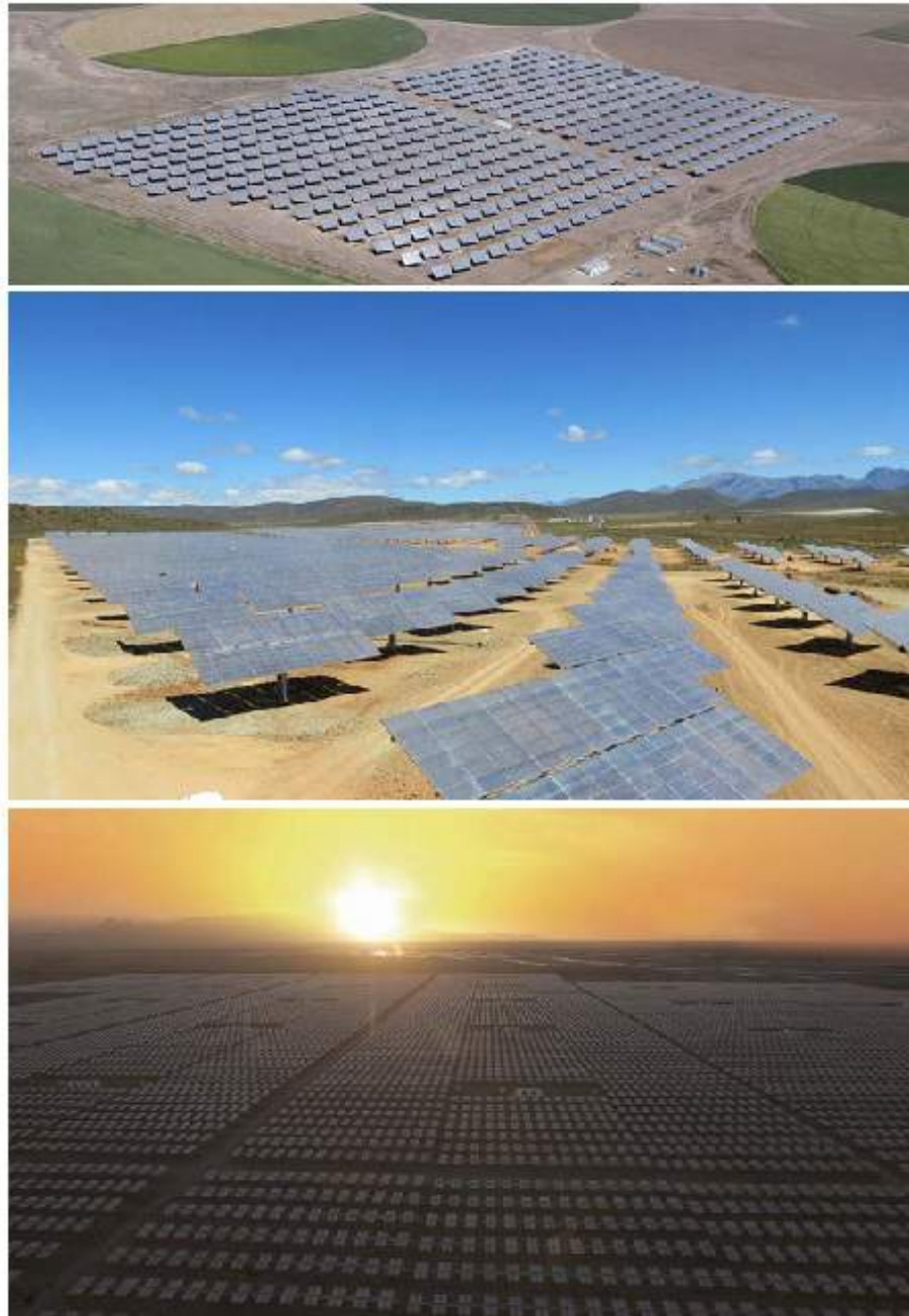
Figure 2.1.1: From top to bottom: 30 MW plant in Alamosa (Colorado) by Amoniz; 44 MW in Touwsrivier (South Africa) by Soitec; 140 MW in Golmud (China) by Suncore. By Fraunhofer ISE [12].
