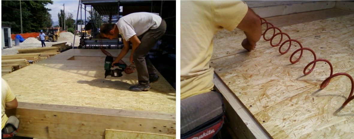
Figure 3-85 Pre-assembly of prefabricated Light-Frame walls.
