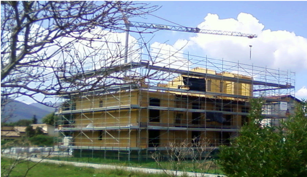
Figure 3-83 Three story residential building for social housing built near Lucca, Italy.
