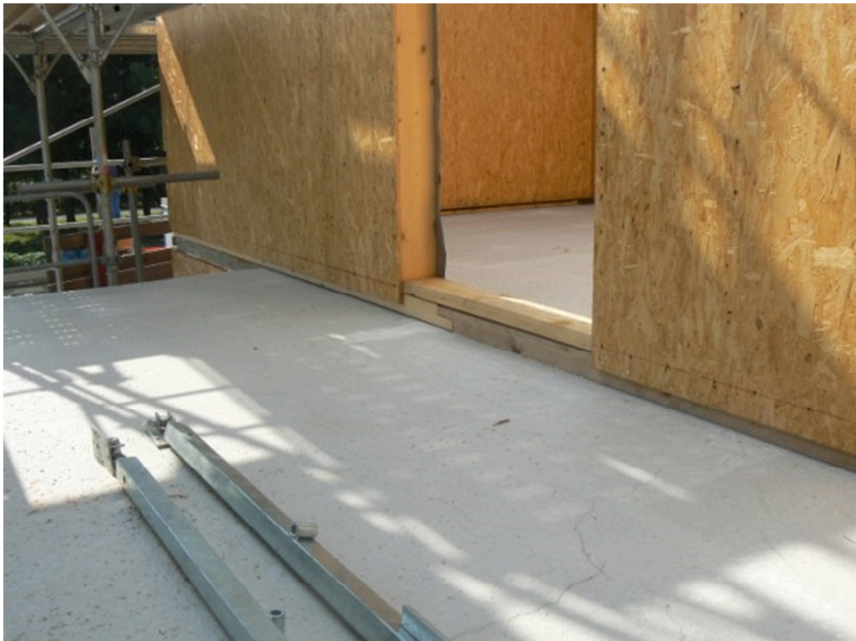
Figure 3-87 Timber-concrete composite floor construction in Light-Frame building.
