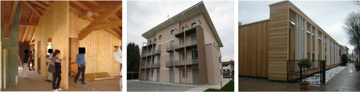
Figure 3-2 Internal view of the structure of a 3-story residential CLT building (left), completed 4-story CLT residential building (center) and completed CLT school (right).
