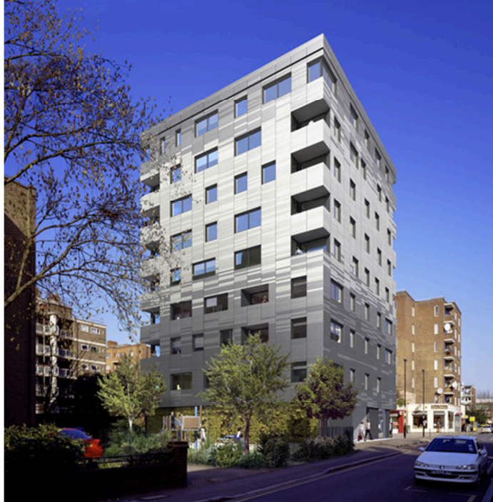
Figure 6-1: Nine storey CLT building built in London in 2008. Structures were built in nine weeks. Design: Waugh-Thistleton Architects.
