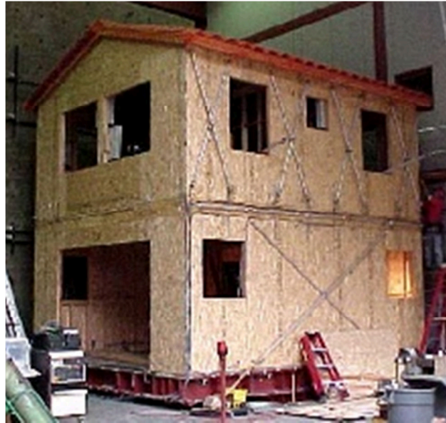
Figure 3-104 View of the test building over the shaking table (after Fischer and Filiatrault, 2000).
