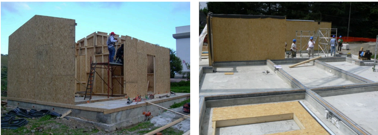
Figure 3-92 Different type of Light Frame erection procedure: walls assembled directly on the building site (left) and assembly of prefabricated walls (right).
