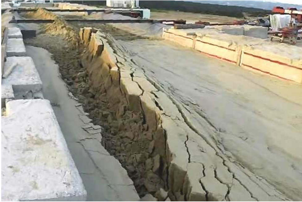
Fig. 145. Soil deformation occurred for 3290 mm of central caisson displacement, Test No. 9.
