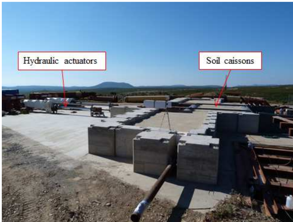
Fig. 6. Testing equipment for landslide/fault experiments.
