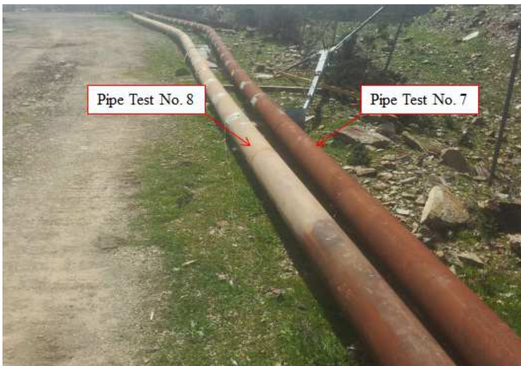
Fig. 134. Pipe final deformation after the Test No. 7 and Test No. 8.
