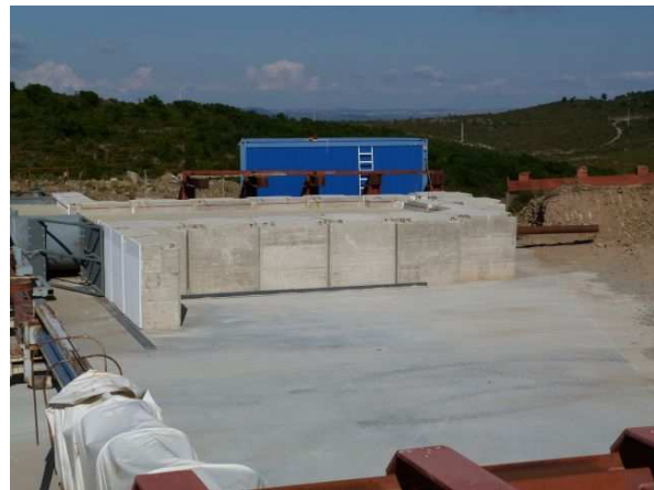
d). Fixed right caisson.
