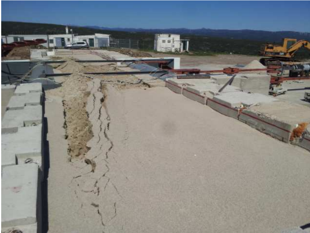
Fig. 133. Soil deformation occurred for 3200 mm of central caisson displacement, Test No. 8.
