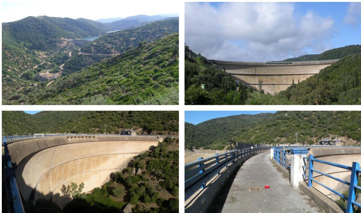
Figure 6.2: Some pictures of Punta Gennarta Arch Dam.
