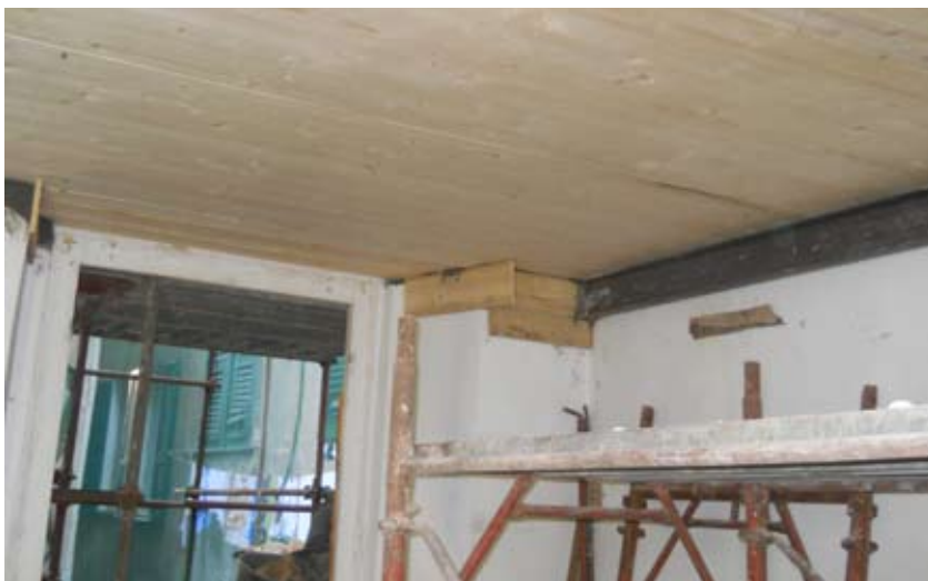
Fig. 18. Solaio in X-LAM in Via S.Bernardo 7.
