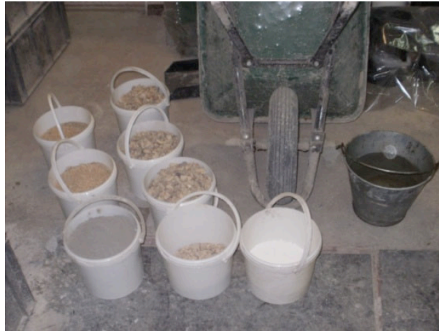
Figure 5.4: Concrete components ready to be mixed.
