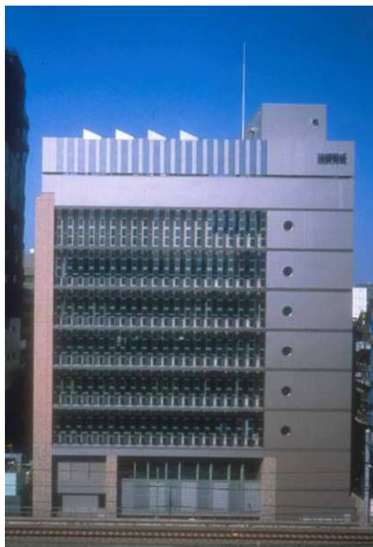
SBIC East Head Office Building, Tokyo, Giappone
