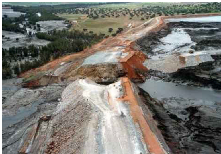
Figure IV.4 Escaping of water from a basin of mining waste (by Virotec)
