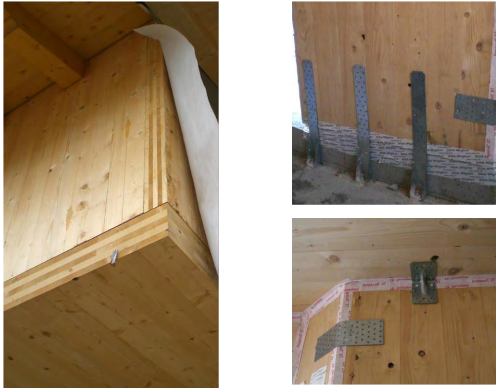
Fig. 4.7 - Example of XLAM construction system.
