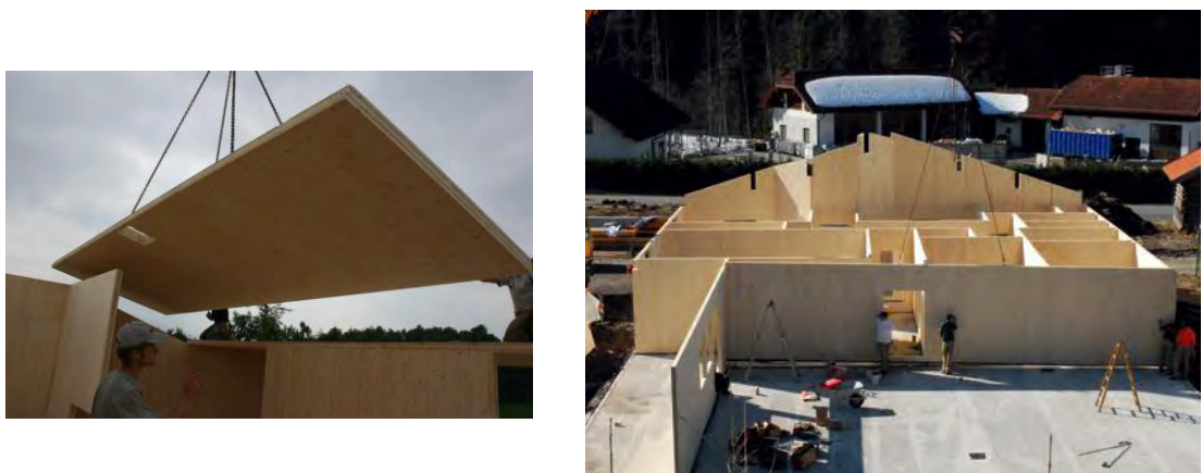
Fig. 4.8 - On-site erection of a XLAM building [Stora Enso Timber].
