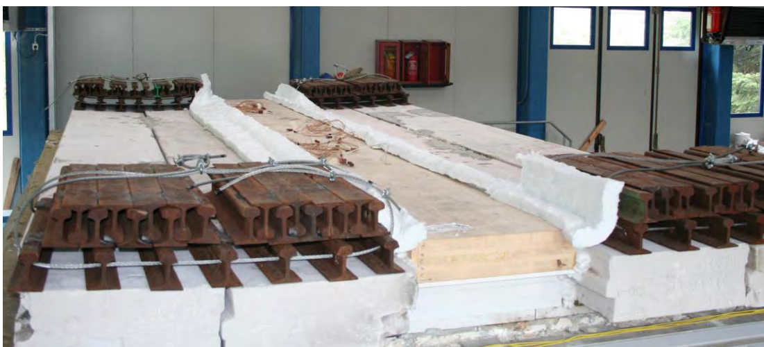
Fig. 5.12 - Setup of large-scale fire tests No. 1 and No. 2.
