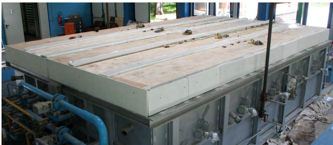
Fig. 5.14 - Setup of large-scale fire test No. 3.
