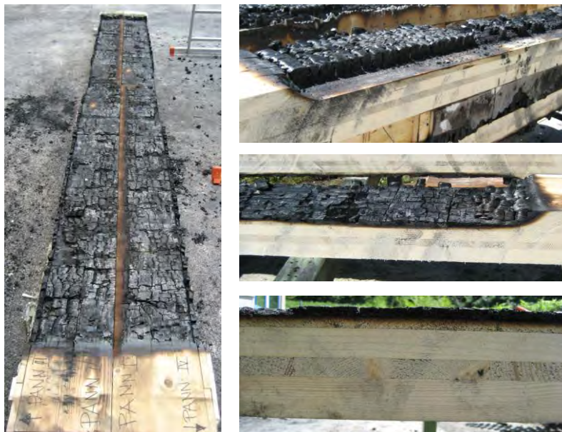
Fig. 5.32 - Unprotected specimen S3-I after fire exposure.
