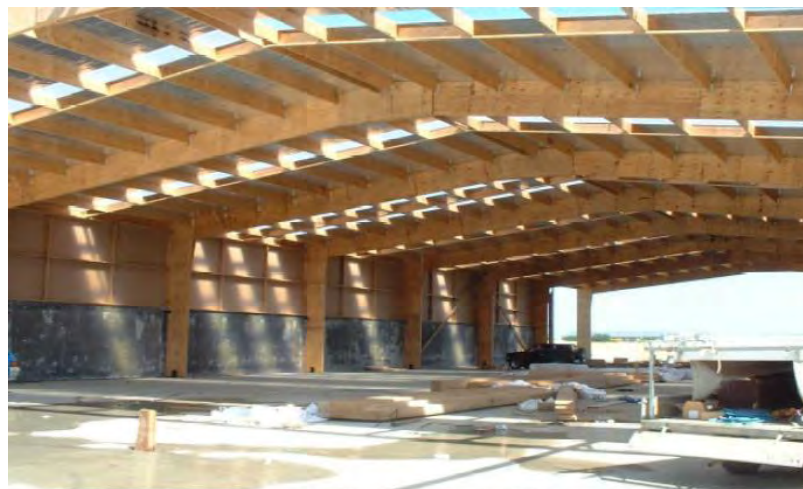
Fig. 1.4 - A LVL portal frame in New Zealand [CHH Woodproducts New Zealand].
