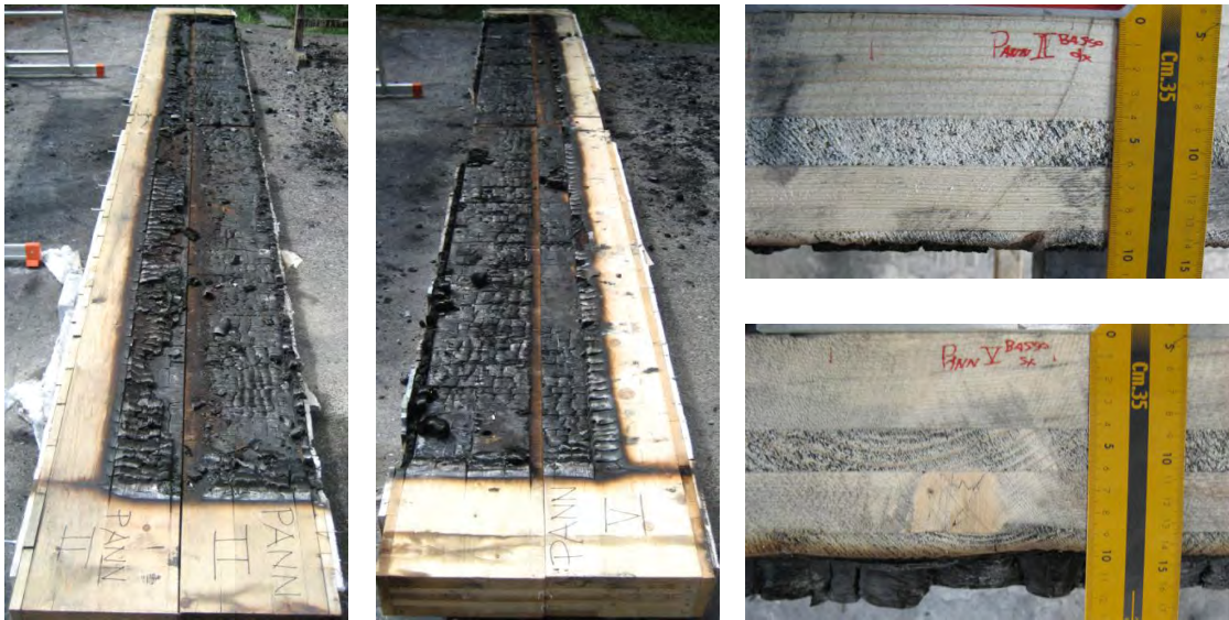
Fig. 5.33 - Unprotected specimens S3-II and S3-V after fire exposure.
