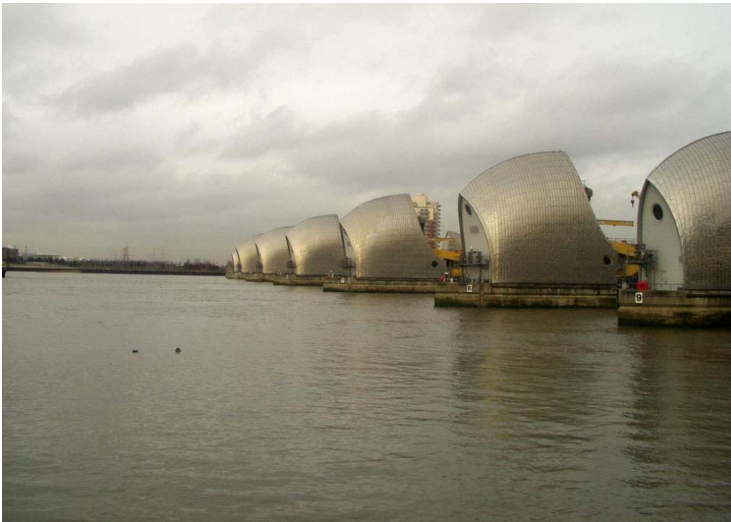
Figure 6.2: The Thames barrier
