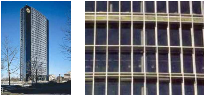
Figure 2.4: Shaft Box (Dusseldorf, ARAG 2000 Tower) - http://gaia.lbl.gov/
