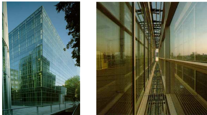
Figure 2.8: Multi Storey Facade (Cologne, Victoria Life Insurance Building) - http://gaia.lbl.gov/
