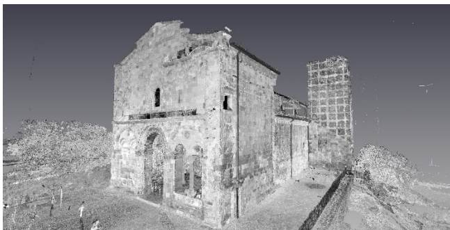
Fig. 5. Aligned pointcloud produced by the 3D Laser Scanner, external view of the Cathedral.
