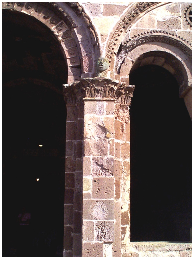
Fig. 2. Worked and squared pyroclastic ashlars in left side of the bifora in main façade of the Cathedral.
