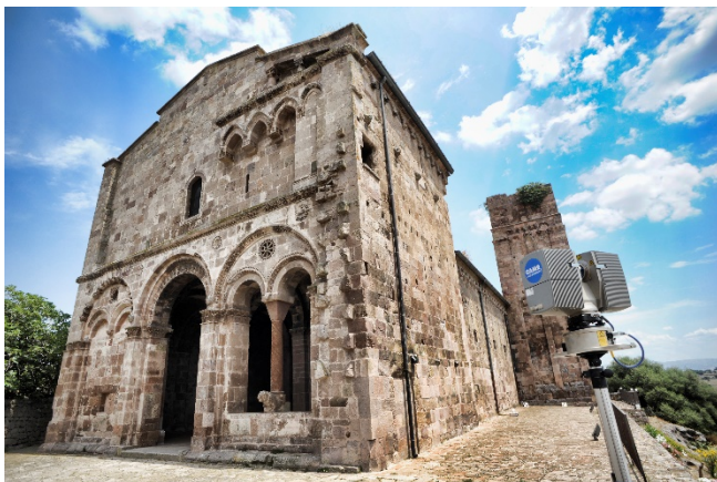
Fig. 1. The 3D Laser Scanner at work along the perimeter of the Church.
