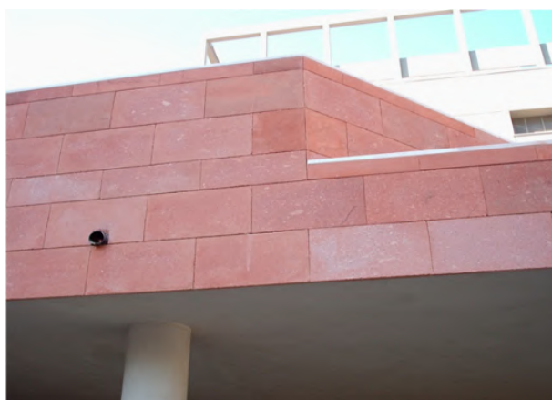
Figure 10. A detail of Teatro Massimo in Cagliari; the cladding, installed following a “run” pattern with runs in variable heights, was built using Fordongianus red “trachyte” (renewed in 2009).
