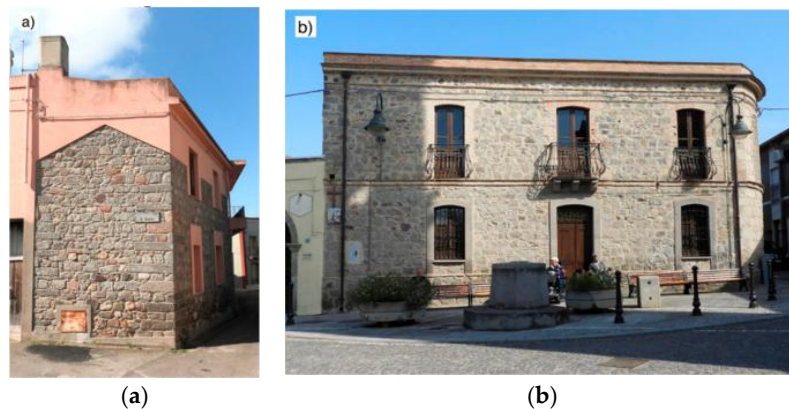
Figure 5. (a) and (b): two examples of houses, (a) and (b), built by using “Pietra di Serrenti”.
