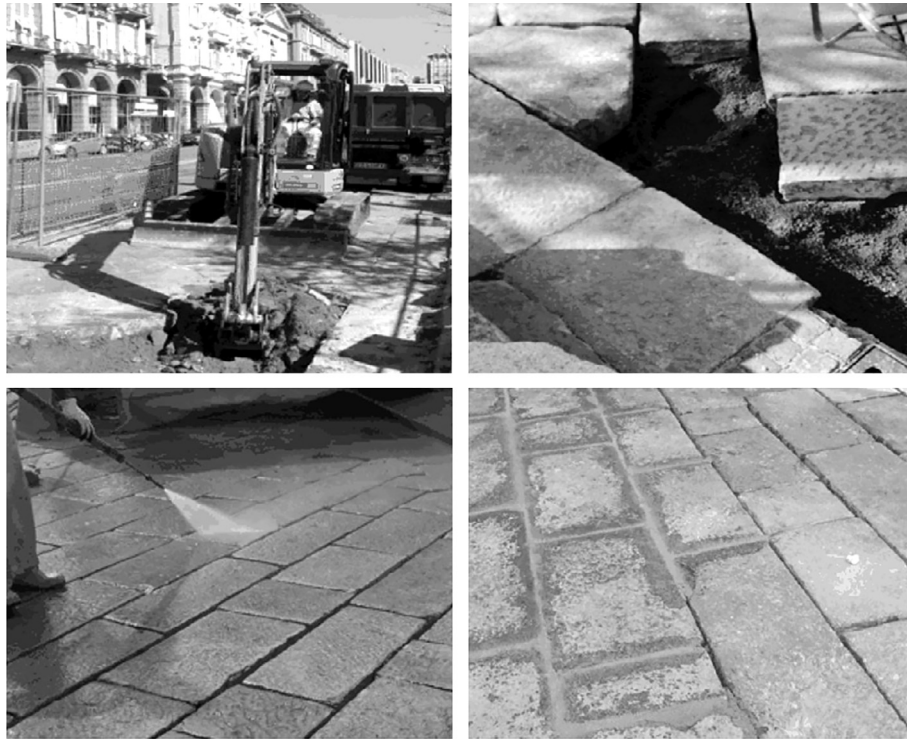
Fig. 5. Removal of the cement-sand deteriorated layer, cleaning, and joint sealing.
