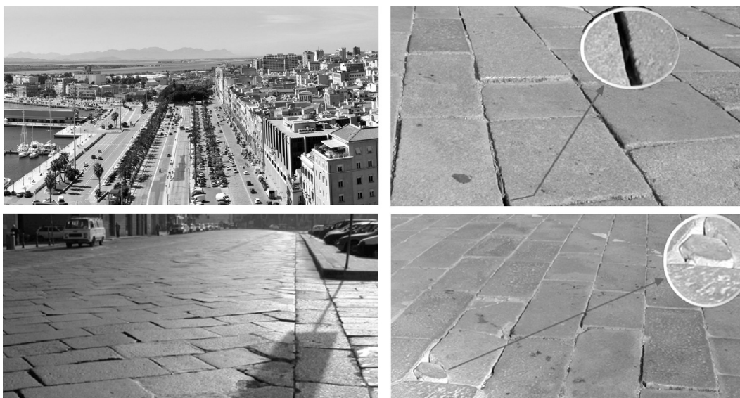
Fig. 2. The flagstone pavement on the Cagliari waterfront and typical distress.
