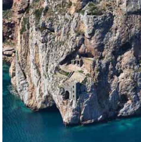
Fig. 08 : The system of terraces that connect the mouths overlooking the sea, of the loading and unloading tunnels, photo by Gianni Alvito, Archivio Parco Geominerario Sardegna
