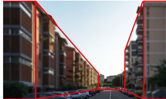
Fig. 1. Example of a real flat roof bidimensional urban canyon in the city of Cagliari (Italy).
