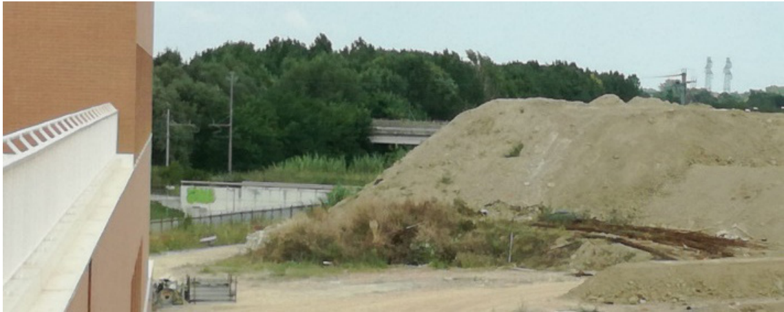
Fig. 6.3: The artificial hill created to protect the building from pollution coming from the railroad and the highway.
