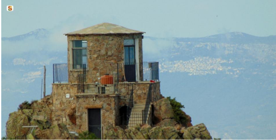
Figure 7. Fire lookout “Montiferru” Cardedu (NU). Author: Giovanni Lotto, image downloaded from www.sardegnaforeste.it
