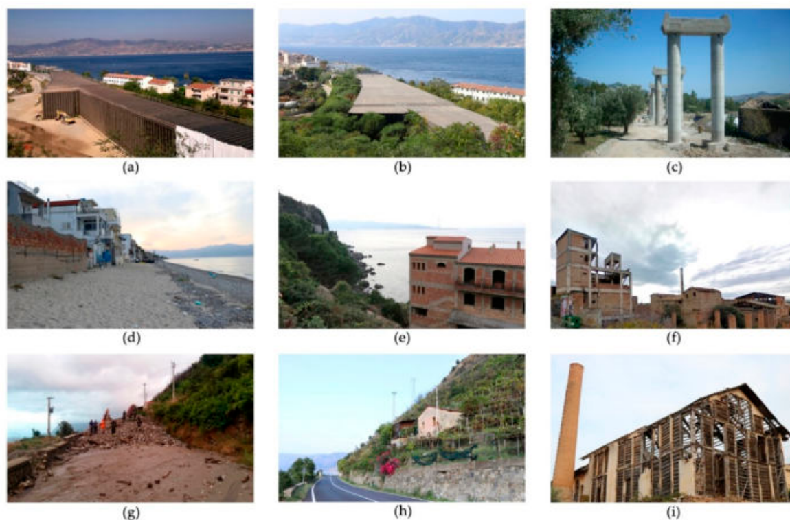
Figure 5. (a,b) Variant of the Cannitello-Villa San Giovanni railway line, preparatory work for the start of construction of the Bridge over the Strait, never built; (c) modernisation works of Bovalino-Bagnara, a transversal artery connecting the Mediterranean Motorway to the SS 106, never completed; (d,e) abusive or abandoned building near the Tyrrhenian coast; (f) Aspromonte wood processing inactive plant of the XIX century. The buildings have industrial archaeology restrictions imposed by superintendence; (g,h) a collapsed terrace due to the abandonment of crops, then recovered and recultivated; (i) abandoned spinning mill of the XIX century.
