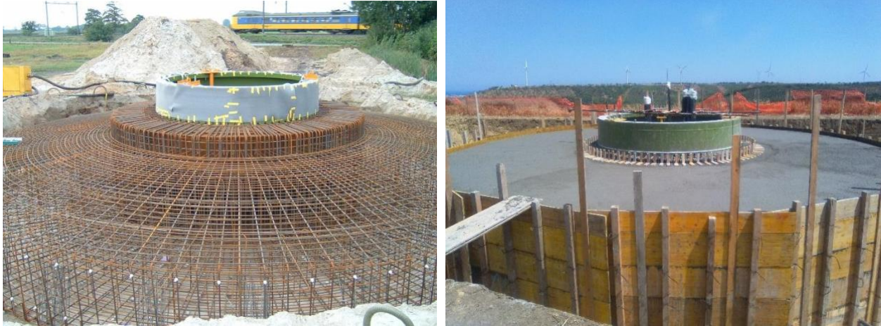
8 9 Figure 2. Example of concrete foundation for onshore steel turbine: reinforcement rebar 10 arrangement (left) and concrete block (right).
