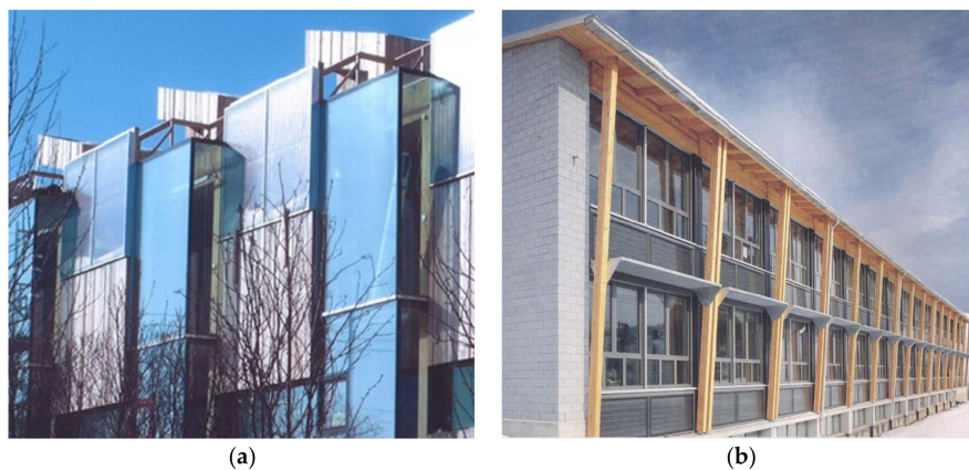
Figure 3. Integration on façade with glazed flat plate collectors: (a) residential complex in Storelva-Tromsøe and (b) school building in Geis, Switzerland.
