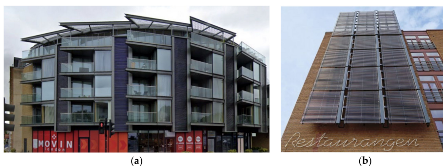
Figure 4. Integration on façade with vacuum tube collectors in residential buildings in London (a) and Malmö, Sweden (b).
