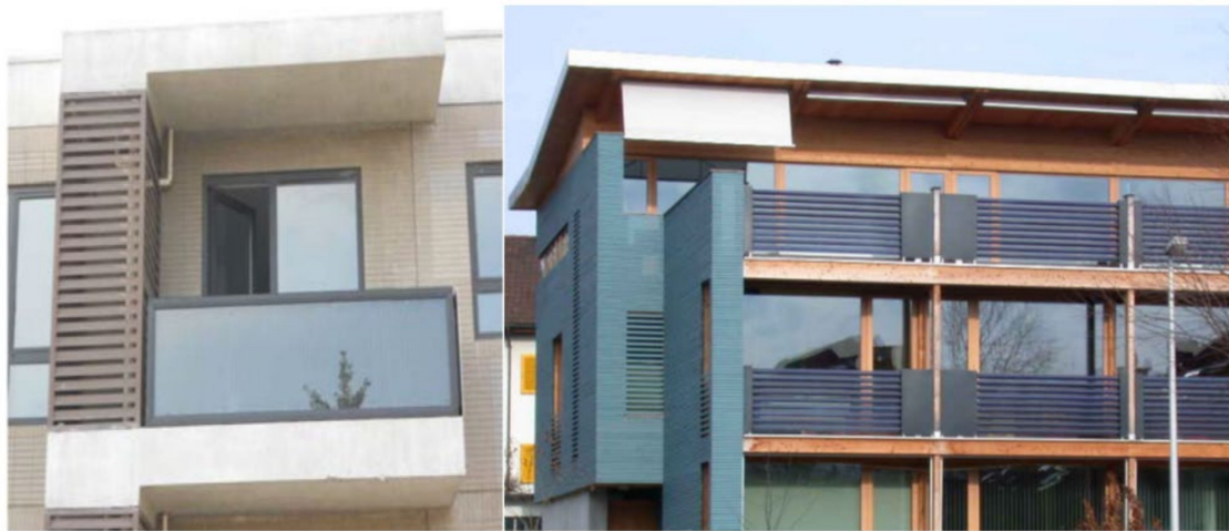
Figure 7. Glazed and evacuated tubes collectors used as balcony balustrades.
