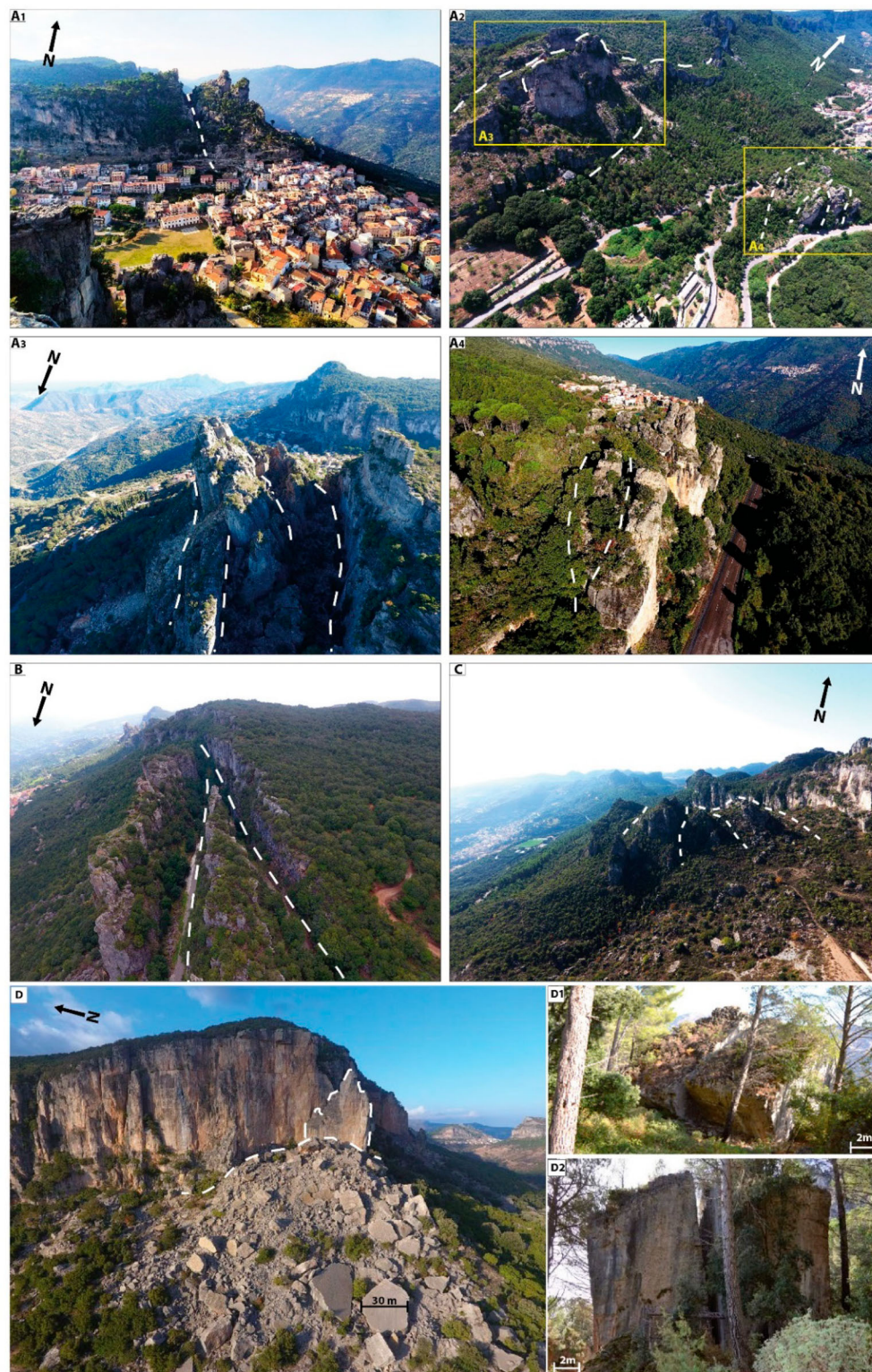
Figure 6. UAV images of the DSGSD showing the major geomorphological and structural features. The white dashed lines represent the major extensional trenches. (A1). Panoramic view of the Ulassai Village. (A2) Brunco Pranedda DSGSD. (A3) Top slope sector. (A4) Middle slope sector. (B) San Giorgio DSGSD. (C) Tisiddu Mountain DSGSD. (D) Evidence of collapse deposits of rock avalanches. Recent collapse near Ulassai Village. (D1, D2) Palaeo-collapse of mega-blocks, 20–40 m for each side.
