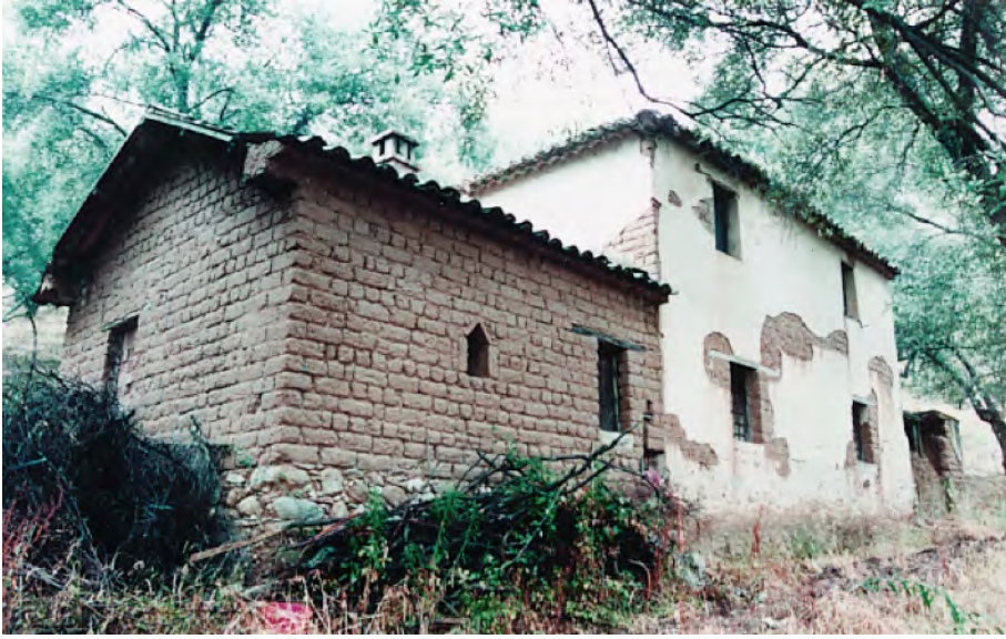
Fig. 5 Calabria, Rural Houses. Credits: R. Chimirri
