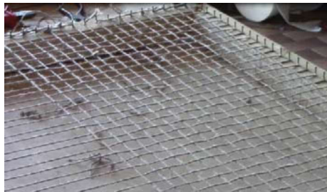
Figure 2: Detail of the on-site fabrication of hemp mesh.
