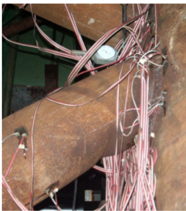
(a) Bulge at the end of the compression brace of specimen CFST-6
