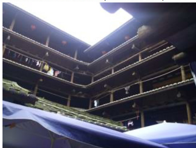
Figure 6. Inner view of the wood structures of a square tulou
