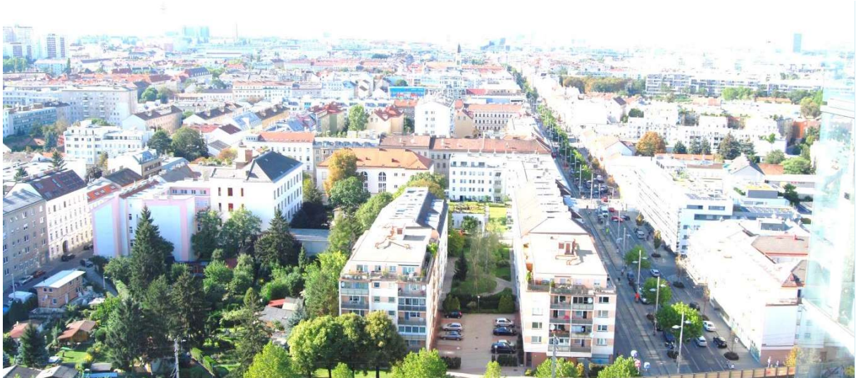
Fig. 2 - Simmering, social housing area in Vienna (source:project Smarter Together)
