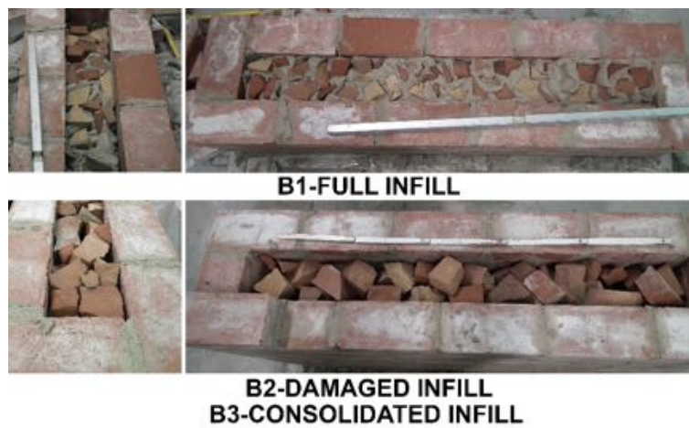
Fig. 2. Construction phases of masonry specimens.
