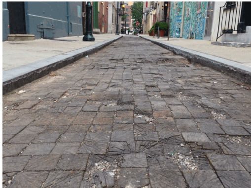
Figure 1. South Camac street (Philadelphia, USA) was paved in wood in 1917 and restored in 2017. It is an example of “Nicolson pavement” still exists in several Countries
