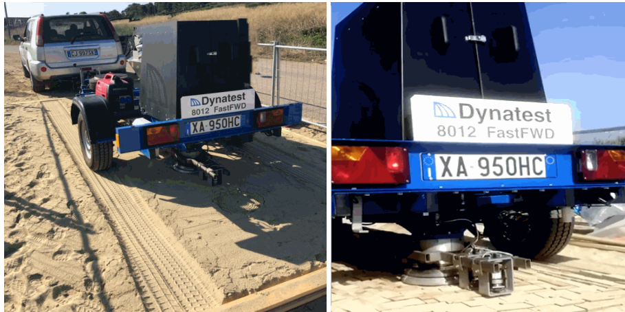
Figure 6. Performing FWD tests on the pavement trial section
