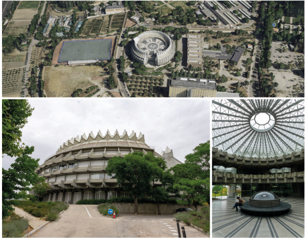
Fig. 3. The current building housing the IPCE (sources: top, Bing Map; bottom, photographs by S. Cera).
